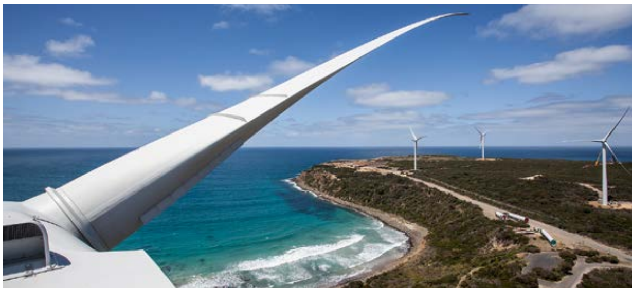
Portland wind farm © Pacific Hydro
