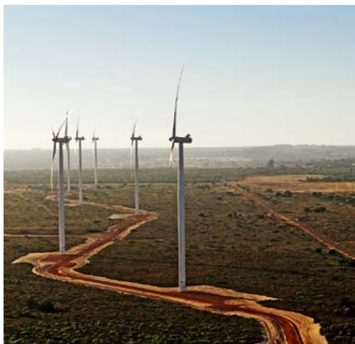
Hopefield Wind Farm © Umoya Energy
